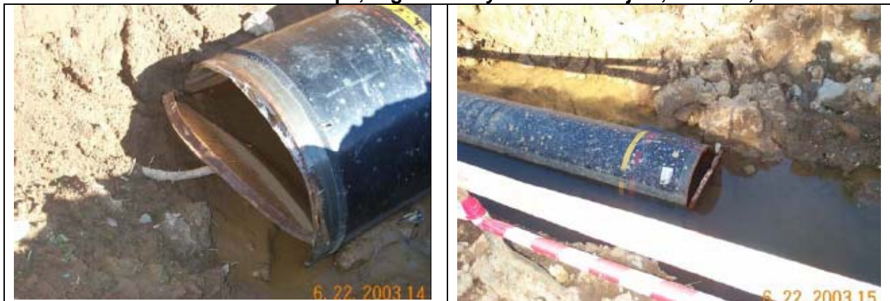
Photos of 14-Inch NGL Pipe, Right-of-Way Camisea Project, June 22, 2003
