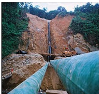
The Camisea pipeline.
